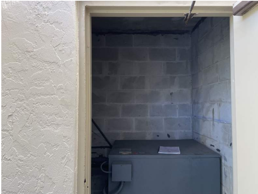
Figure 5: Mechanical Room Concrete Masonry Unit Wall
