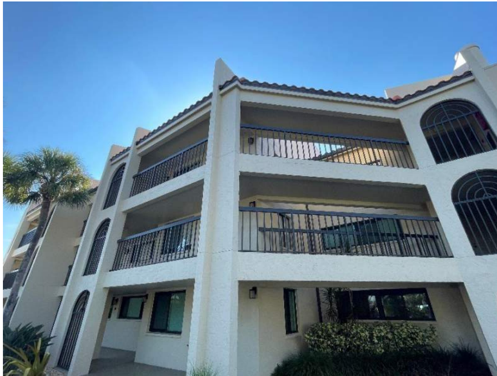
Figure 3: Exterior Concrete Columns
