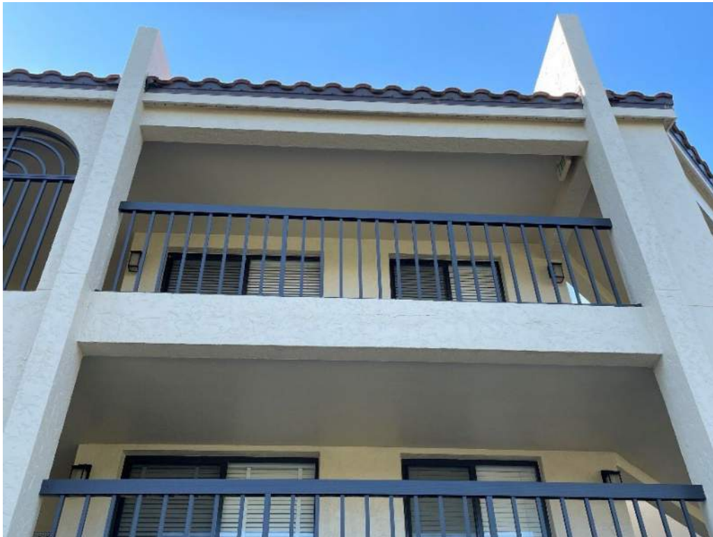
Figure 4: Exterior Concrete Beam
