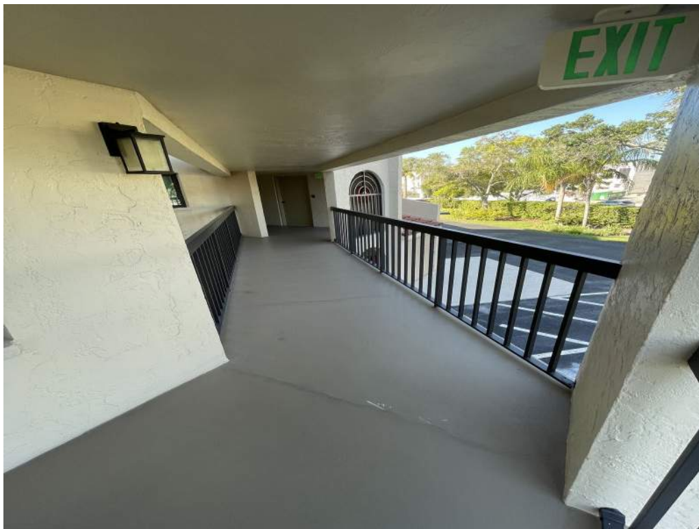
Figure 6: Exterior Concrete Walkway Slab
